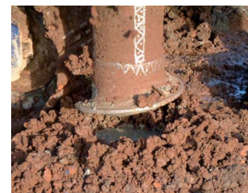
A concreted pile — No spoil to dispose of.
